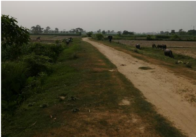
Earthen access road to reach the subproject site
