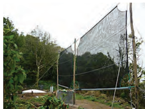
Fig. 3-5 Fog Collection System Source: http://www.fogvest.org
