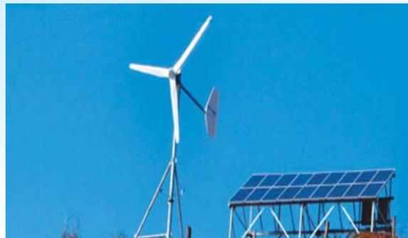
*Wind Solar Hybrid System (Wind generators and Solar panels)*
