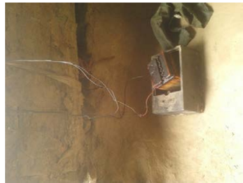
Fig. 4.5: Systems with Damaged Battery/Control Box
