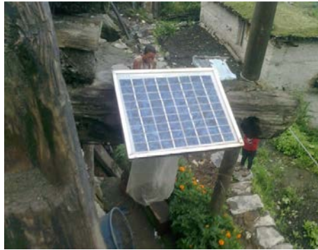
Fig. 4.1: An Example of Well Installed Module
