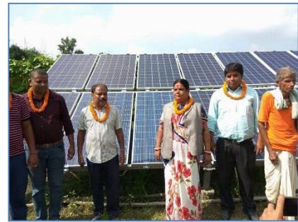
Minister visits Telkuwa PVPS Project
