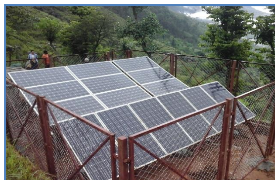
Rehabilitated Solar Panel house
