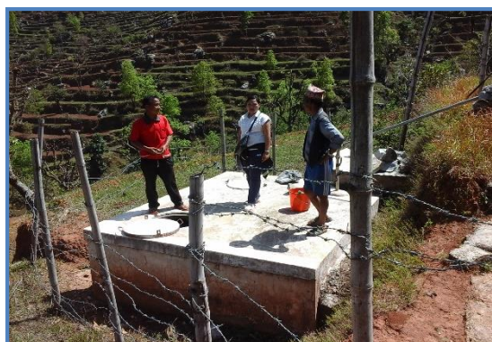
Water collection tank before rehabilitation
