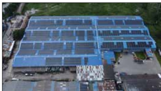
Figure 11: Solar Rooftop installed with support from AEPC/KFW-DKTI Solar Project
