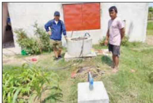
Figure 17: Domestic Biogas Plant installation
