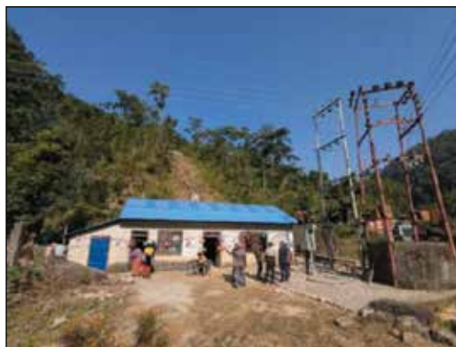
Figure 7: Jhumsa Khola III Grid Interconnected Micro Hydro Project (68 kW), Mathagadhi Rural Municipality, Palpa
