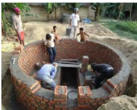
Biodigester wall (under construction)
