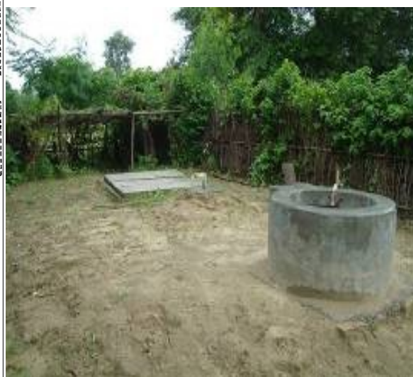
Fig: Biogas Digester in Operation
